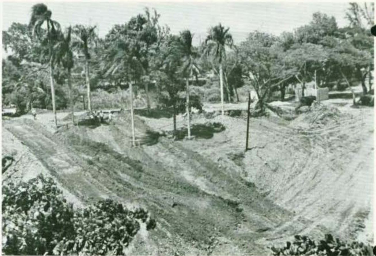
Work in progress on the chapel and religious center.
