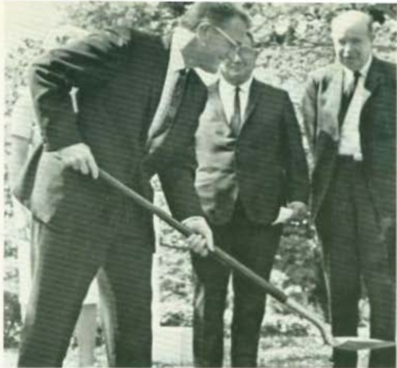
Dr. Hoxeng takes his turn with the shovel at the groundbreaking ceremony for the Paul A. Wolfe Memorial Chapel and Religious Center. Looking on are Dr. José M. Rodríguez Quiñones, President of the Board of Trustees, and Mr. M. Slade Palmer, Chairman of the Inter American University Committee of the New York Presbyterian Synod. Partially hidden behind Dr. Hoxeng is Mrs. Paul A. Wolfe.
