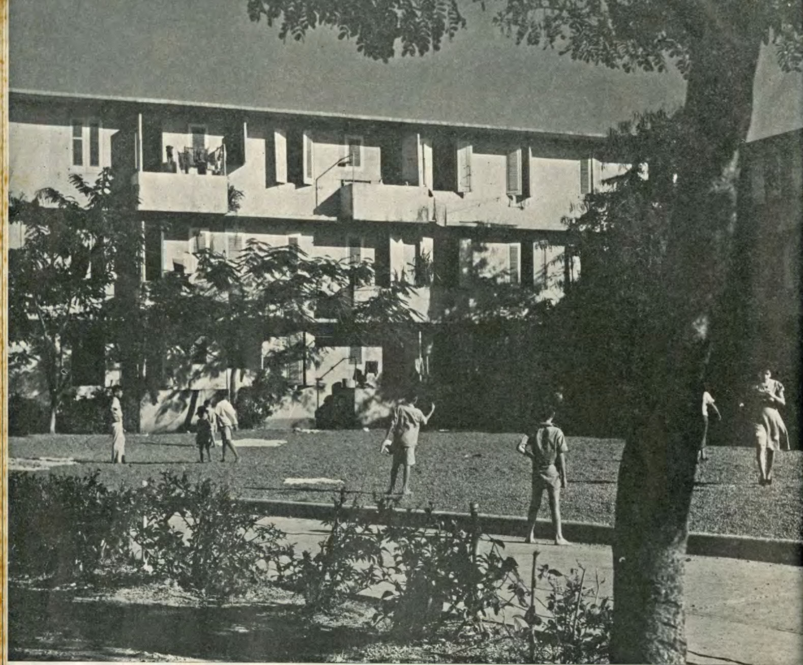
Public housing, halted during the war, is being continued by Federal and Insular Governments. This project was built with Federal funds.
